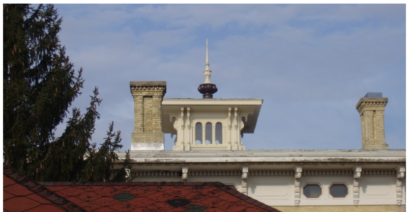
Lincoln-Tallman House Cupola, Restoration Complete
